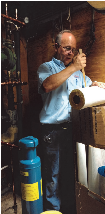
Larry Kastner precisely cuts insulation to wrap the unique system pieces.
